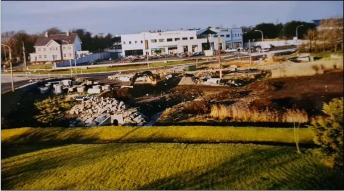
In river works, connecting new roadside drainage directly to the river
